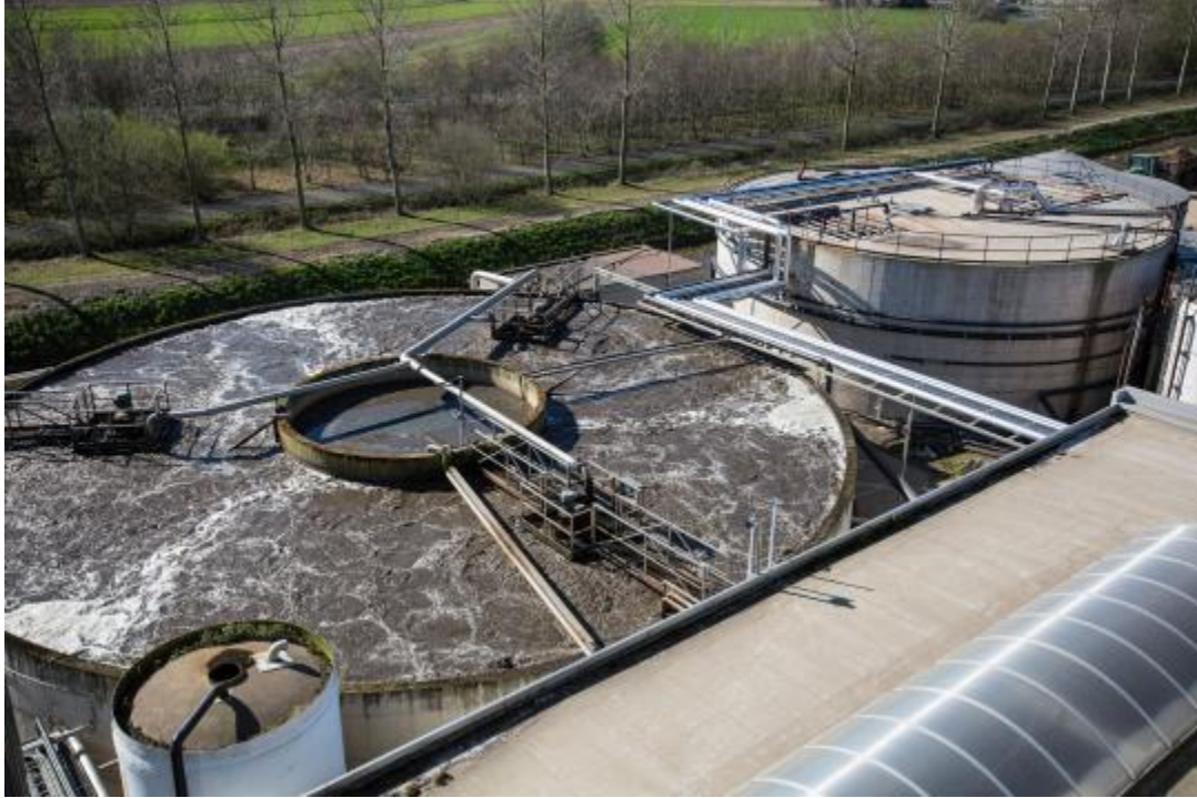
The wastewater treatment plant with the anaerobic reactor (ANUBIX™-B) at the right and the nitrification basin at the left
