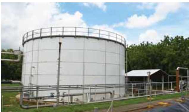
This anaerobic reactor was designed for 24 tons of chemical oxygen demand per day.
