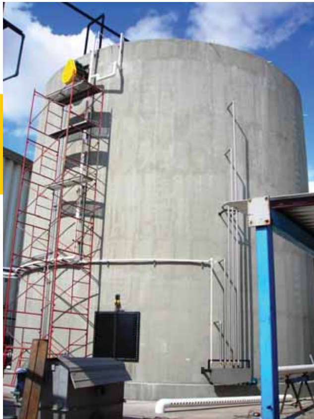
The quantity of biogas to be produced by Sabormex is equivalent to about 2,650 tons of the fossil fuel equivalent per year.
