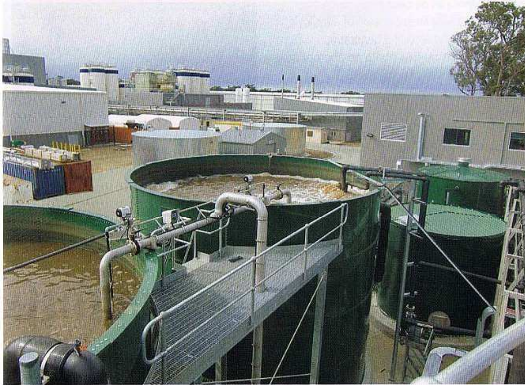
Green power ... the new Bluetongue Brewery in NSW
