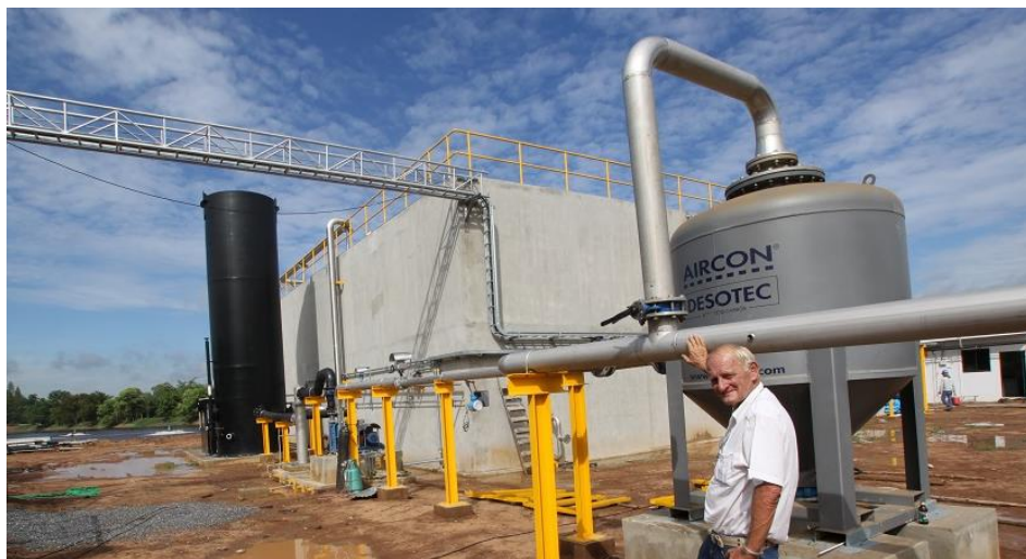
United Farmer and Industry plant commissioning by GWE
