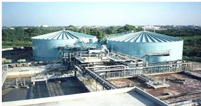
Thai Union Mfg. Wastewater Treatment Plant
