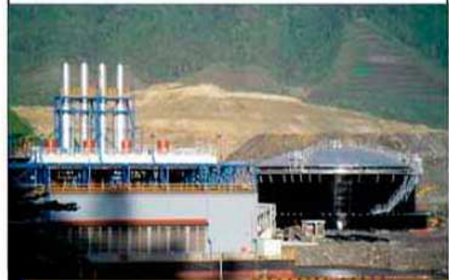
Power Station Project—PNG—Gold Mine
