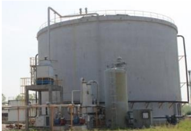
Chok Chai Starch digester and biogas treatment.
