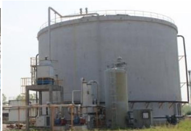
Chok Chai Starch digester and biogas treatment.
